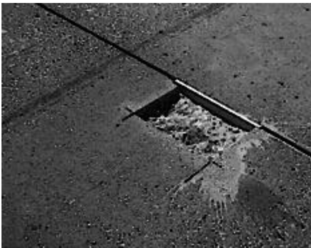
Figure 14. Properly placed compressible insert.
