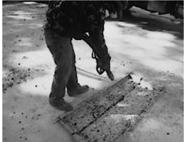
Figure 11. Repair area being cleaned by sandblasting.
