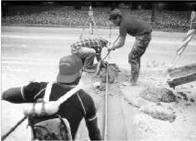
Figure 15. Placing partial-depth repair materials.
