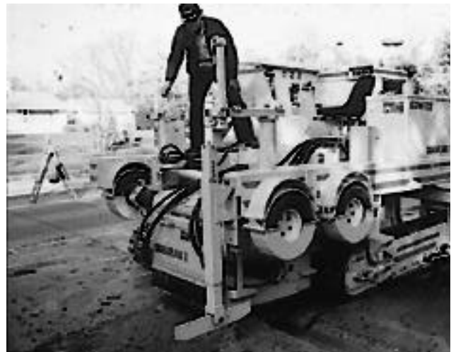
Figure 9. Removal of material within repair area using a cold-milling machine.
