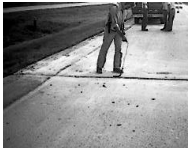
Figure 5. Sounding the pavement with a chain.
