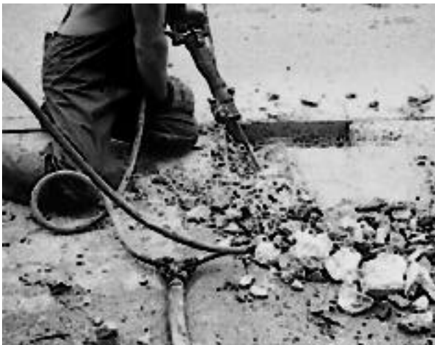
Figure 8. Chipping out the concrete within the repair area.
