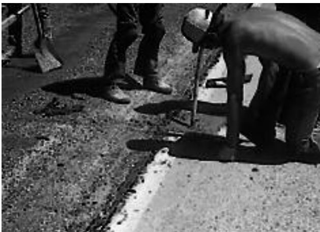
Figure 16. Consolidation of partial-depth repair material.
