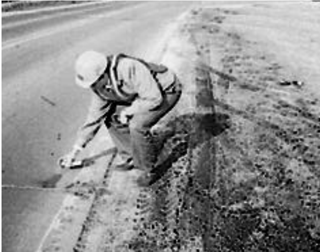
Figure 6. Marking repair boundaries with spray paint.
