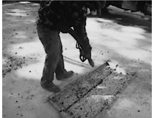
Figure 11. Repair area being cleaned by sandblasting.
