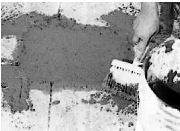
Figure 18. Sealing repair boundaries with cement-water grout.
