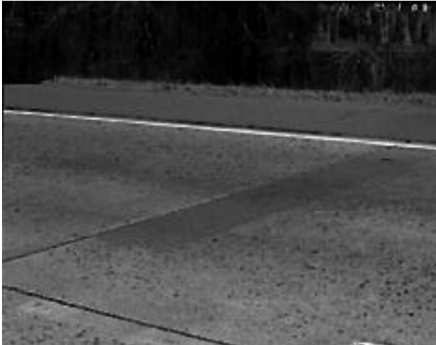
Figure 19. Completed patch after joint resealing.
