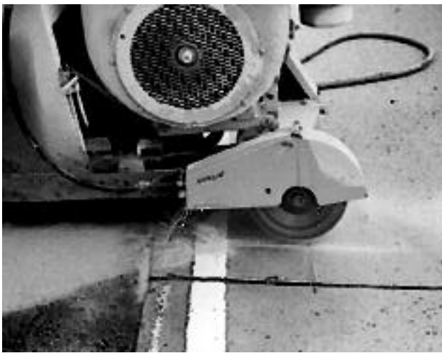
Figure 7. Sawing repair boundaries
