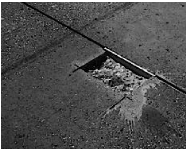
Figure 14. Properly placed compressible insert.
