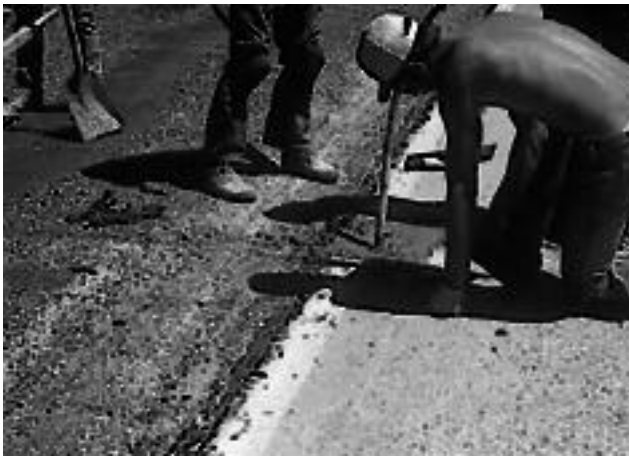
Figure 16. Consolidation of partial-depth repair material.
